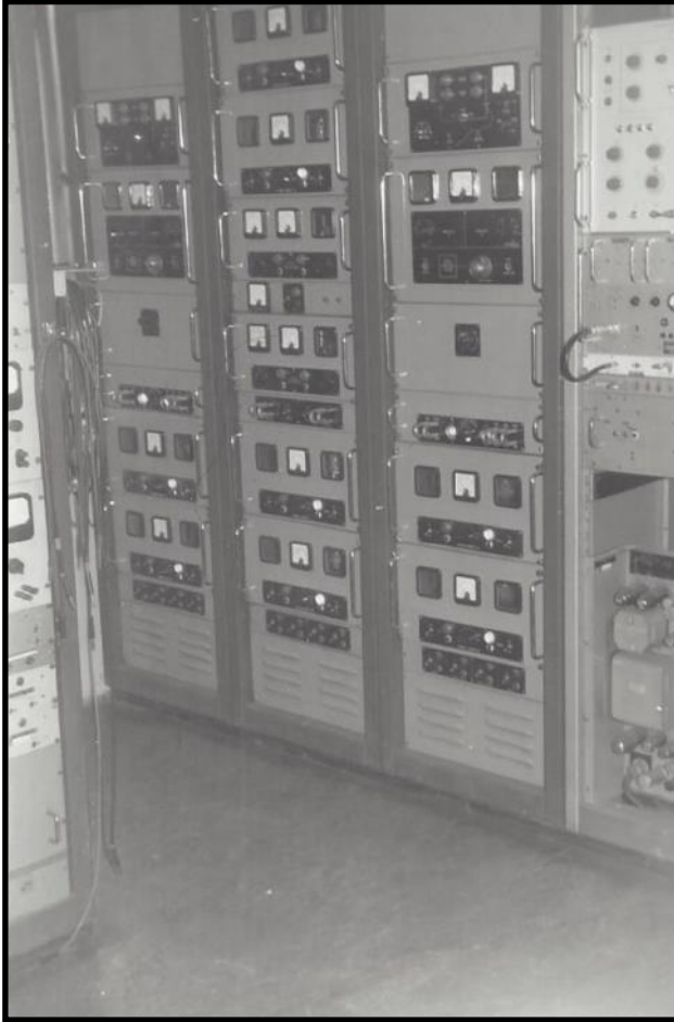
Incoming line processing equipment with Marconi staircase test generator
