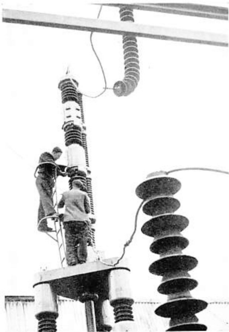
Removing the contacts after the test on the 275 k.v. circuit breaker
