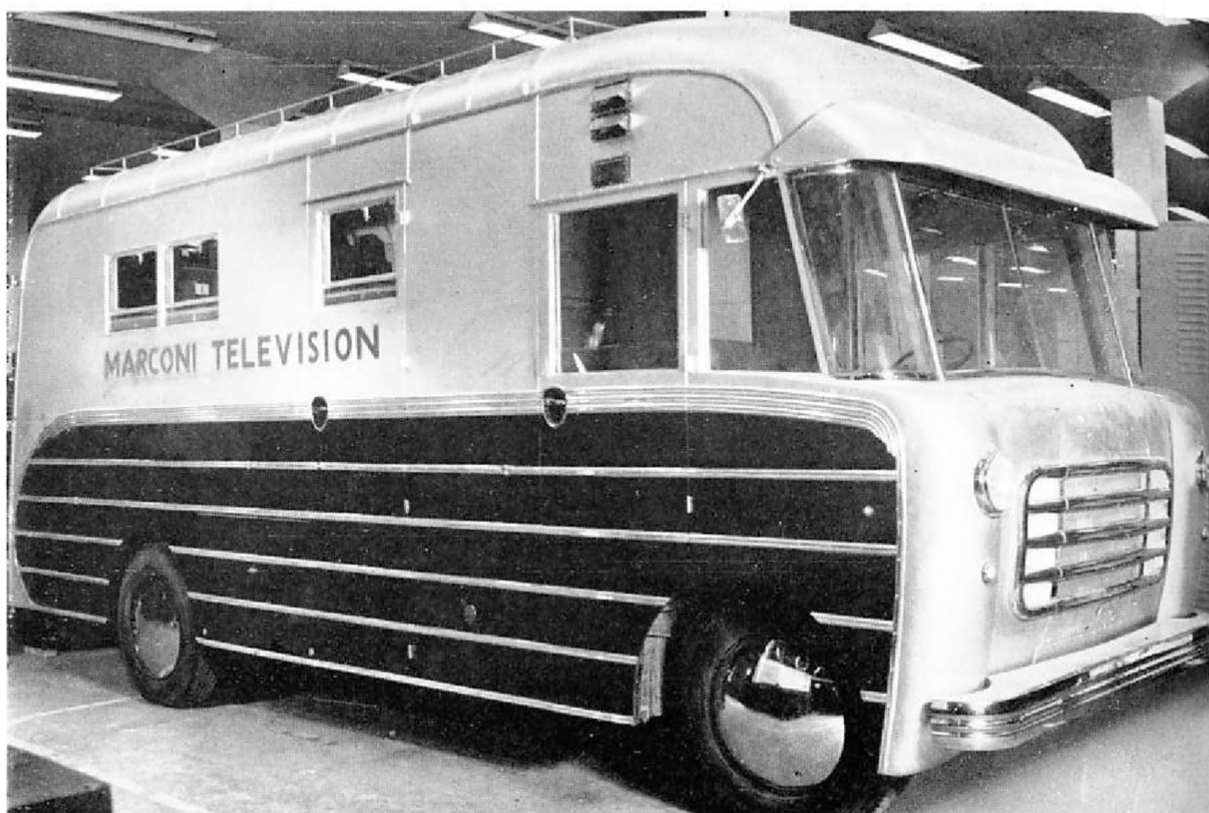
The TV mobile unit van which will be sent overseas to Caracas very soon. On the next page you can see inside. In the foreground is the producer's control desk. The sound mixer is on his left and the mains voltage regulator unit on his right. Beyond are the camera control and the vision mixer units
