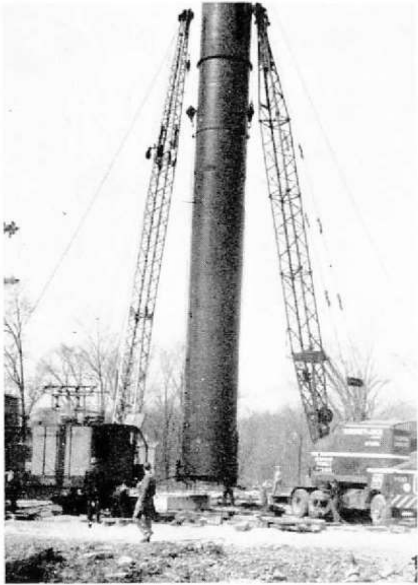
Raising the aerial, which was to carry the finest television broadcast yet produced
