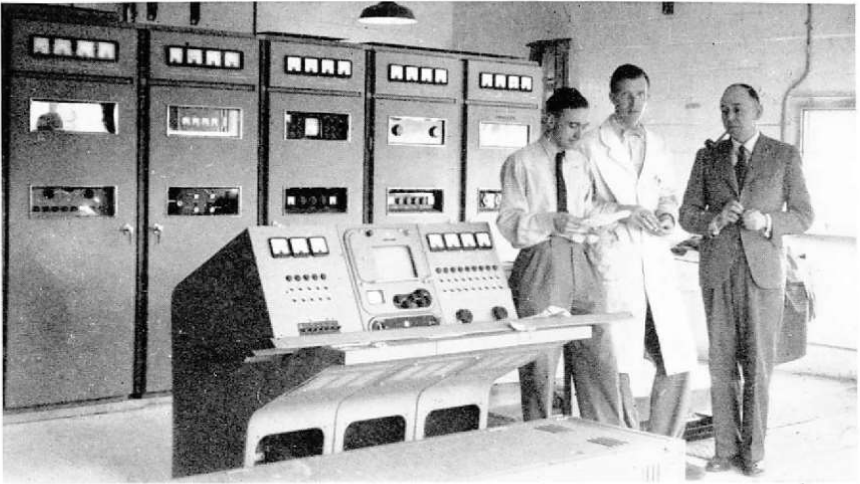
From highly organised chaos emerges the transmitting station. With the set ready for power and testing are G. Williams and D. Lavers, M.W.T., and G. Elliot, C.B.C.
