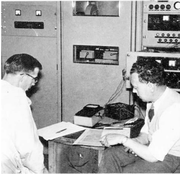
ABOVE: D. Lavers, left, installation engineer, and T. Cooper of Transmitter Development, working on the modulator after the amplifier had been installed
