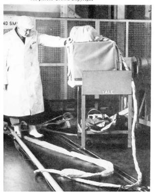
LEFT: Rigged for action in a nylon suit and carrying regulation safety lockets and electroscope is Ron Swinden of this Company's Industrial Television Unit. The entire equipment, with the exception of the camera lens, was covered with protective plastic sheeting
