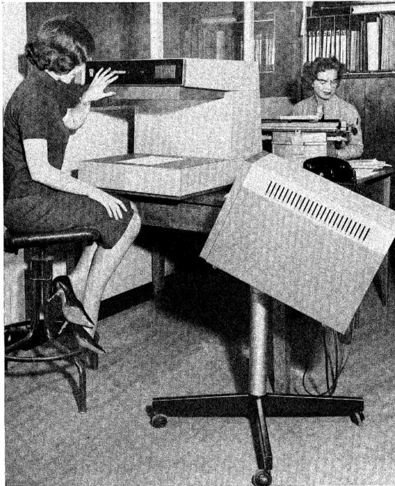
Document transmission equipment.
