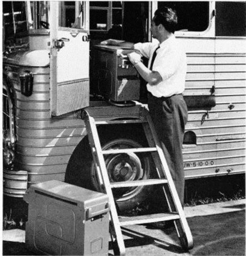
In their mobile form, the camera control and power units are easily handled and are not vulnerable during transit. Adequate handles and a heavy tubular base are fitted.
