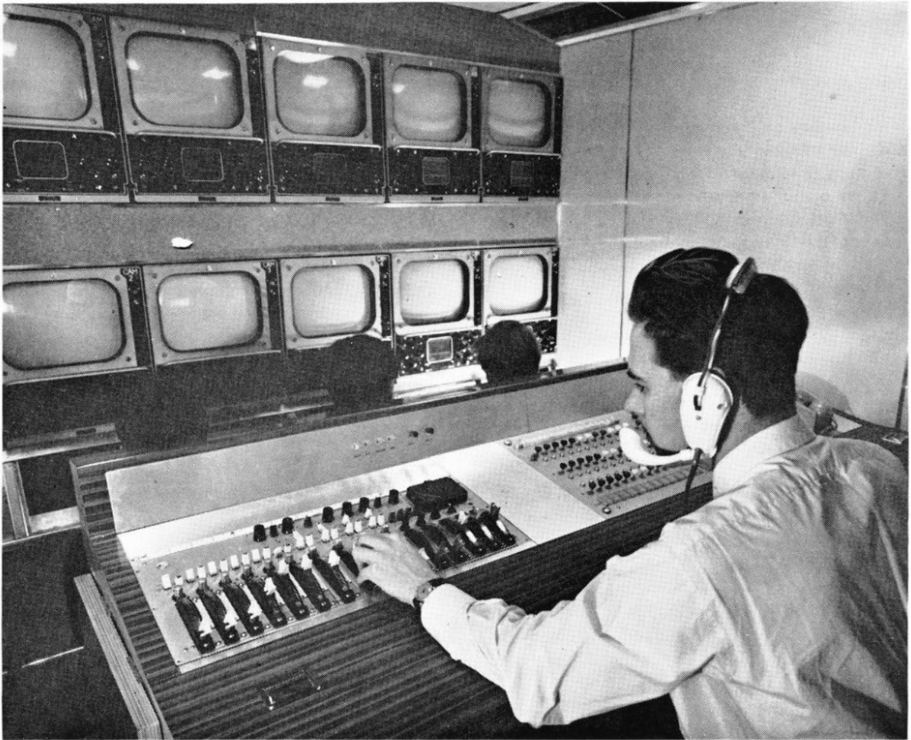
Fig. 3. Interior view showing production area.
