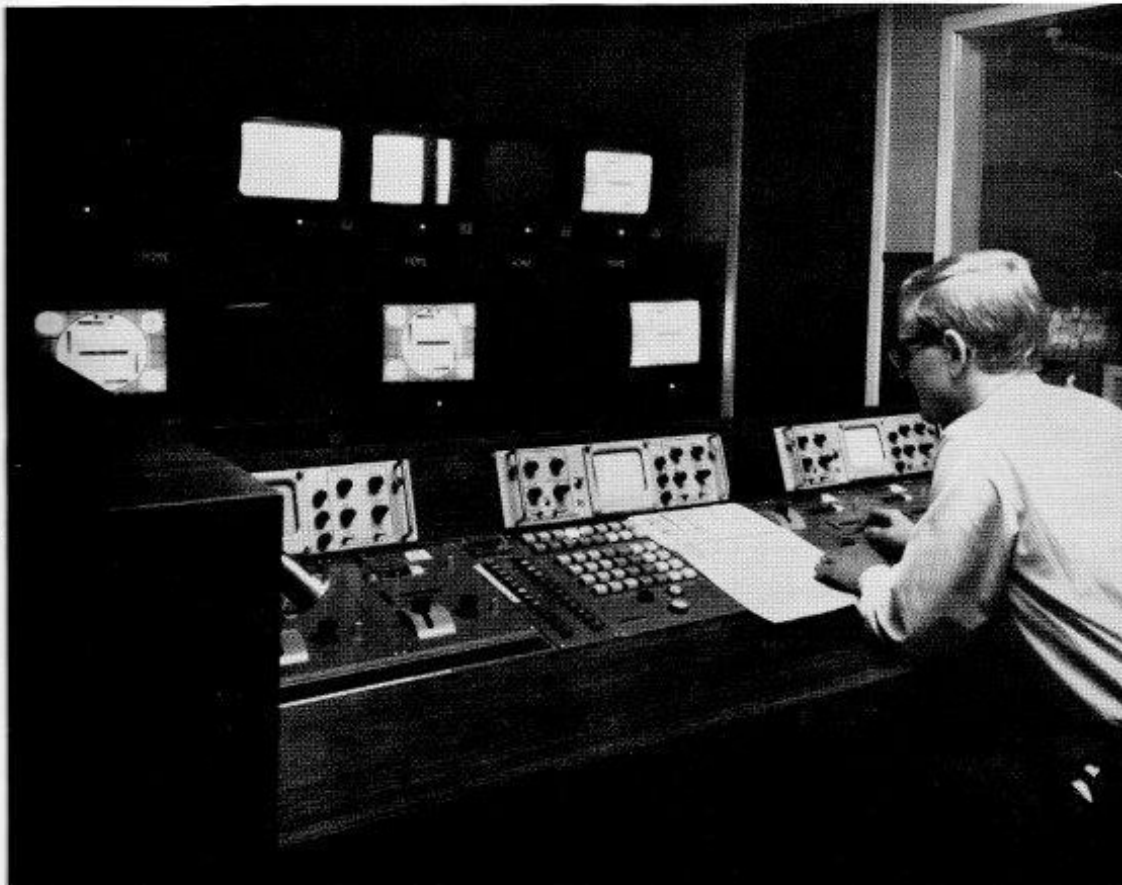
Fig.4 Telecine control and assignment room at Tyne Tees Television. (Tyne Tees picture.)
