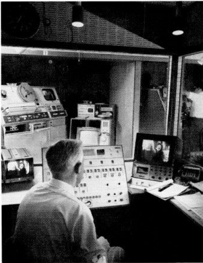
Fig.6 VTR area with VTR assignment control in foreground. (Granada picture.)
