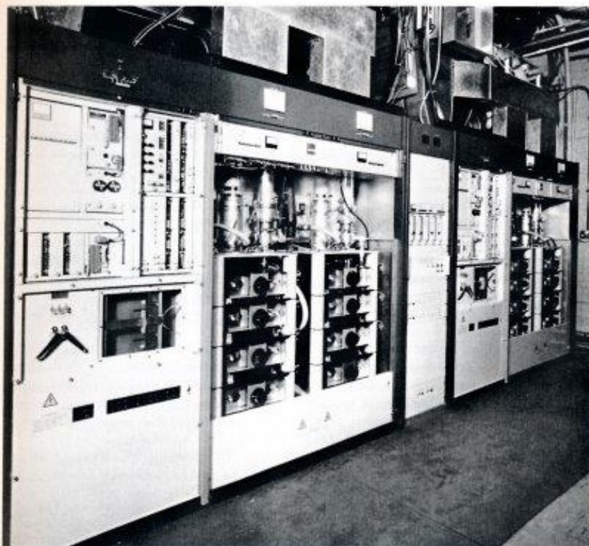
Fig. 7. Front view of a parallel installation of Type B7445 Transmitters
