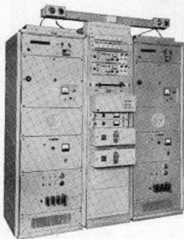
Two unattended 1kW m.f transmitters at BBC Station at Postwick
