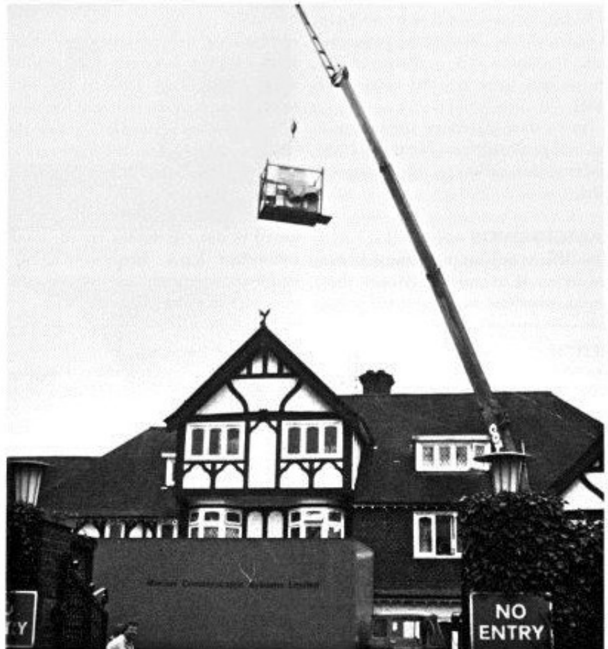
Delivery of the VTRs was complicated by the difficult access at the CTVC premises. They were lifted over the house by crane and lowered, blind, on the far side to a first floor access point.
