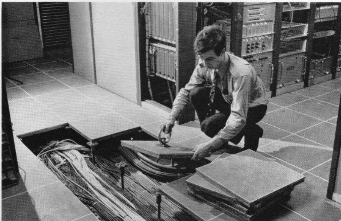
False floors of modular construction using cast aluminium tiles.
