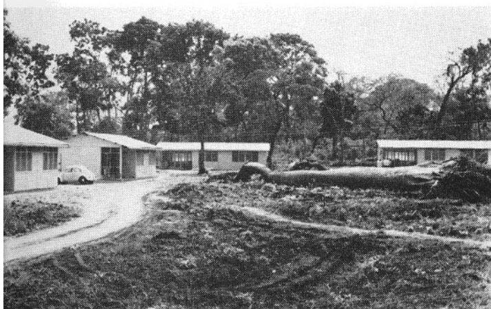
Fig. 8. The temporary bungalows at Ejura which were erected to house the relays of erection teams.
