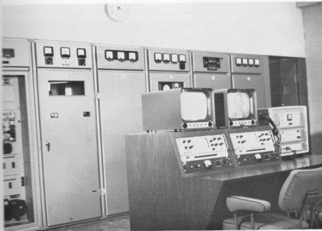
Fig 5 The 10kW Band I vision transmitter and 2kW sound transmitter.
