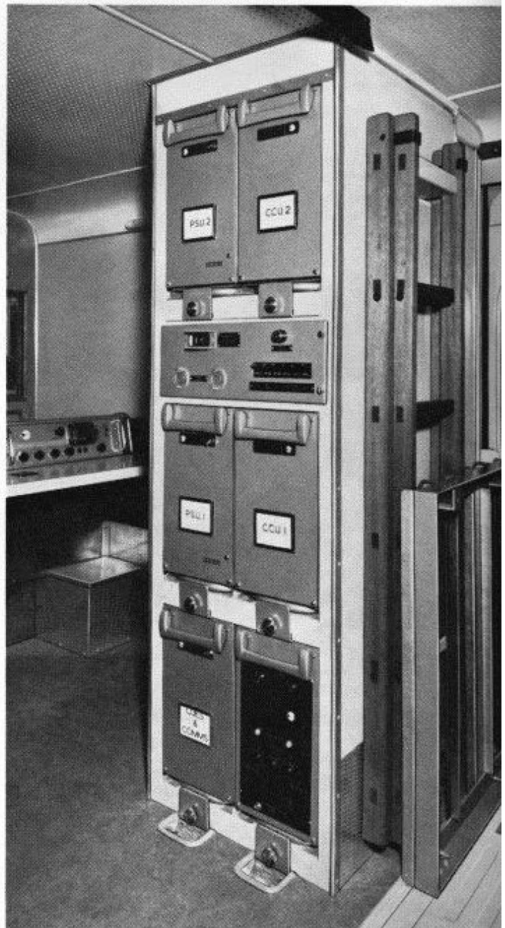
Fig. 2. The equipment rack in the production area, containing the camera control units, power supply units, communication unit and sync. generators.
