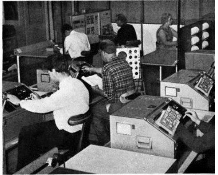
Fig. 2. CCU printed boards on test with semi-automatic a.c./d.c. testers.
