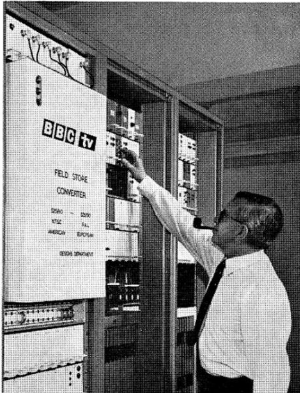
General view of the electronic field store standards converter.
