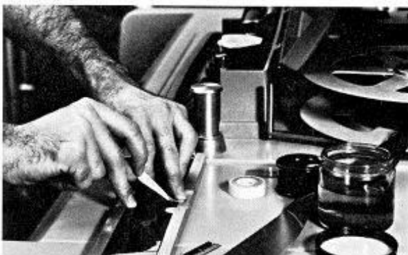
Figure 1. Editing in the late fifties required digital dexterity and splicing tape. The videotape was dipped in a carbonyl iron particle dispersion, which made the edit pulses and the transverse tracks visible. A metal jig, a straight edge and a single edged razor blade was used to cut in the guard band of the verticle interval scan
