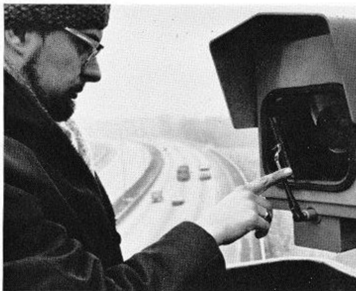
Here is Roger Hobson of E.O.S.D. checking the windscreen wiper on the waterproof housing of the camera. Inside, a small heater ensures that no condensation forms and steams up the optics of the camera
