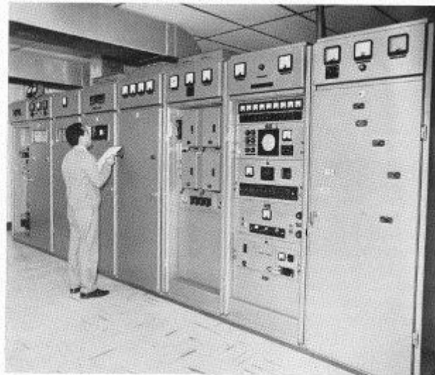
20kW Band III Vision Transmitter type B 7202 and 5kW Sound Transmitter type B 6601 at Channel 13 transmitter hall, Latin American Tower, Mexico City
