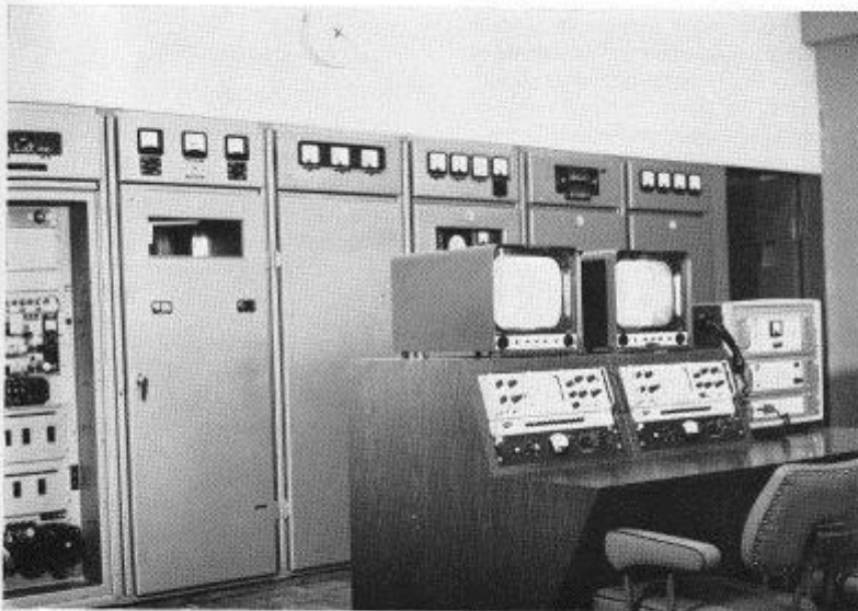
5kW Vision and 2kW Sound Transmitter at Annam, Jordan
