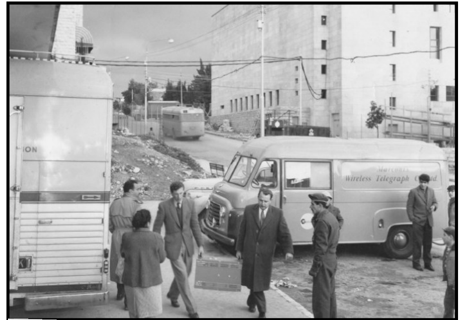
View of the trial building showing our camera cables across the street Terry Barritt and Ron Huntsman unloading equipment from the OB van
