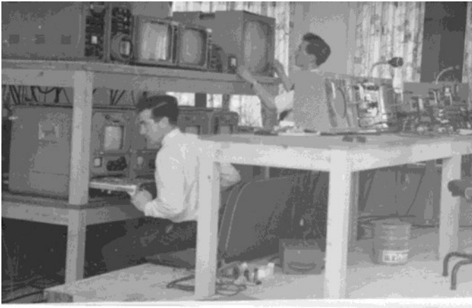
Roy Sharp and Ron Huntsman installing the production system
